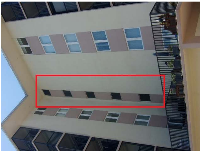
OPENING PROTECTION – Although the unit owner window & sliding door openings are large missile rated, the stairwell windows are not rated or protected.
