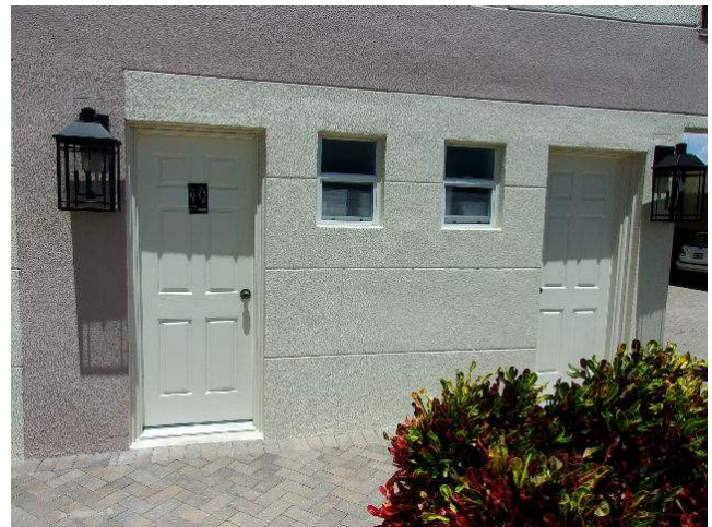
OPENING PROTECTION – The ground level pool bathroom doors are impact rated, but the window units are not rated or protected.
